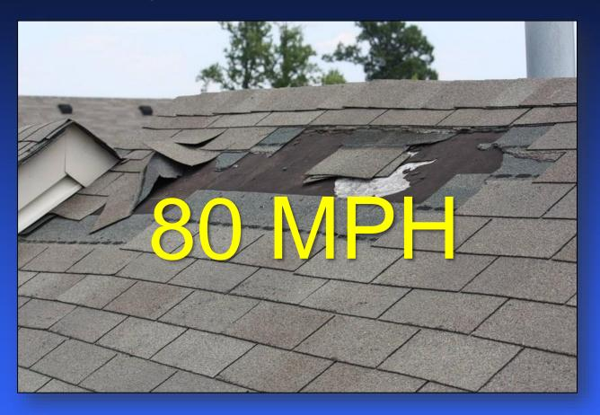
Wind combined weight of water in rain can cause 120 mph rated shingles to fail at a lower wind speed
